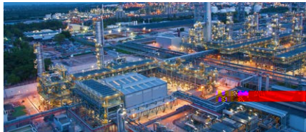
Industrial Park Process Water
